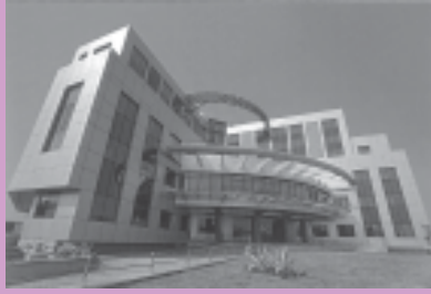
NEW HEAD QUARTERS OF THE INSURANCE INSTITUTE OF INDIA AT BANDRA-KURLA COMPLEX (MUMBAI)
